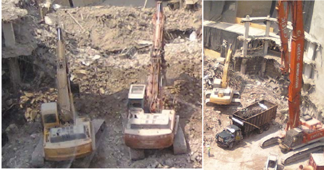
Figure 1- Excavators w/ hydraulic shears
